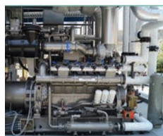
Engines supporting HCTP Cogeneration Plant
