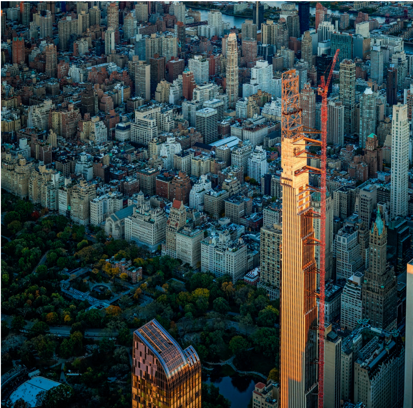
Steinway Tower, at 111 West 57th Street in Manhattan, under construction in 2019
