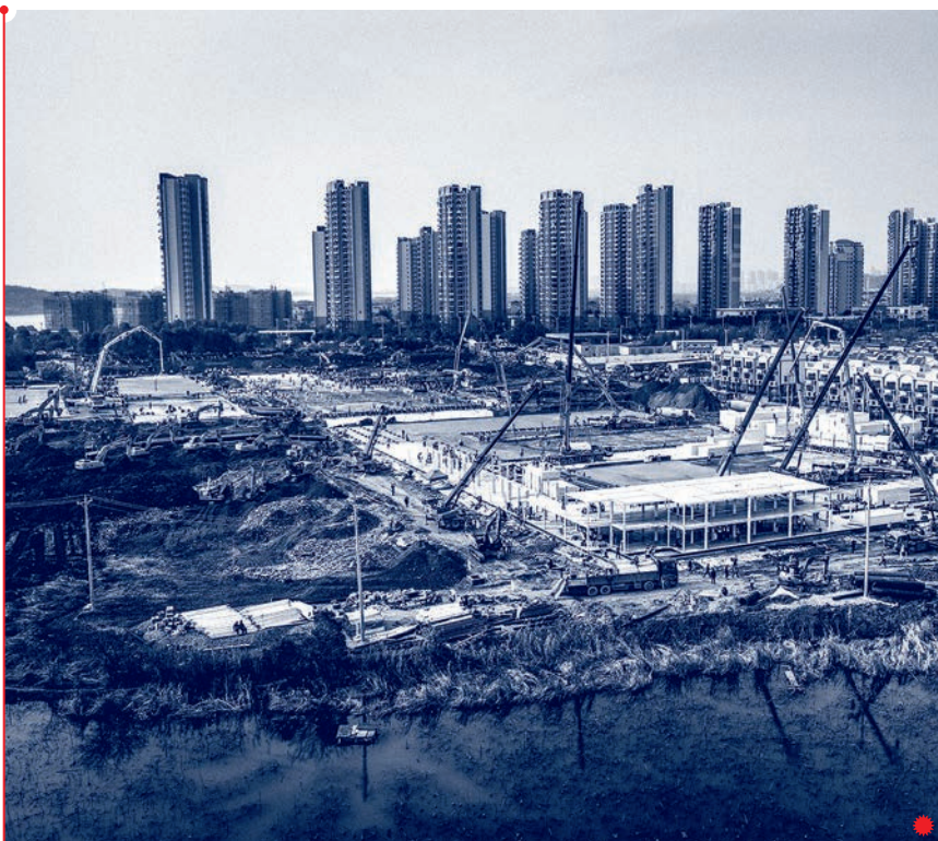
Hundreds of construction workers erect a prefabricated hospital in Wuhan, January 28, 2020.
