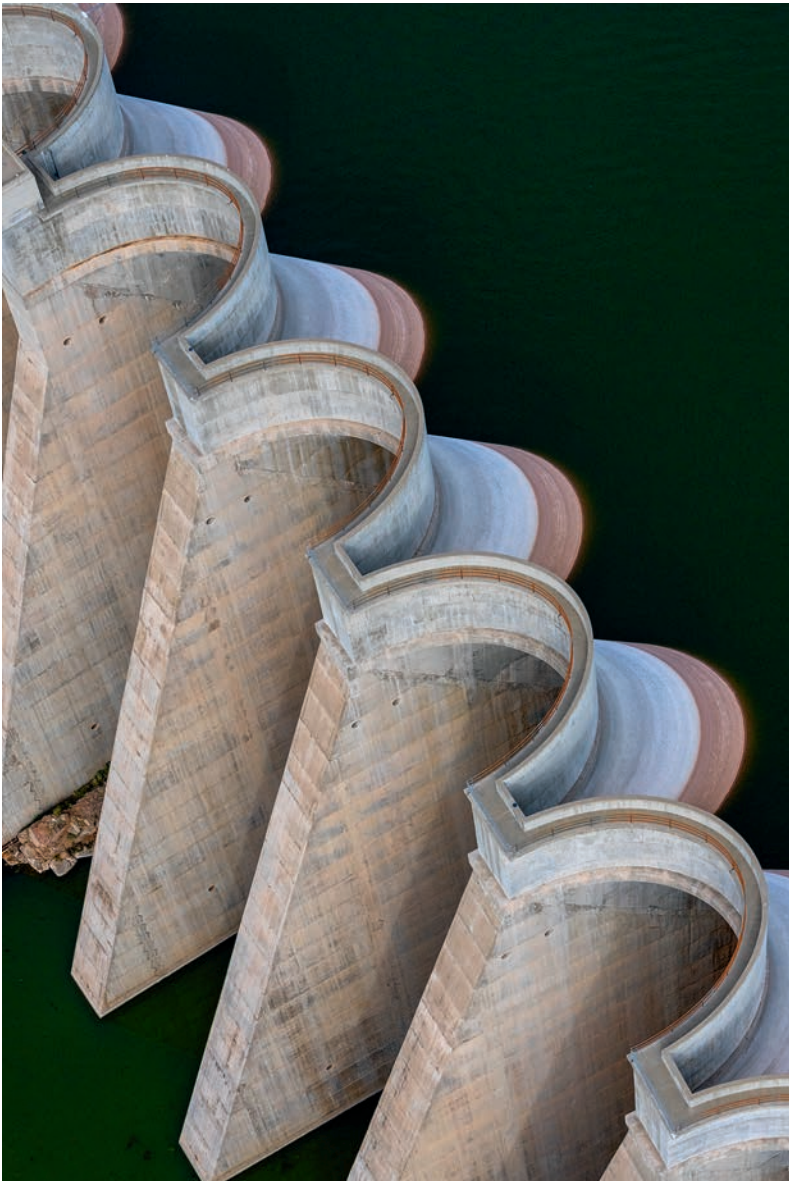
The Bartlett Dam, on the Verde River, is part of the Salt River Project, which manages water allocation in the Valley.
